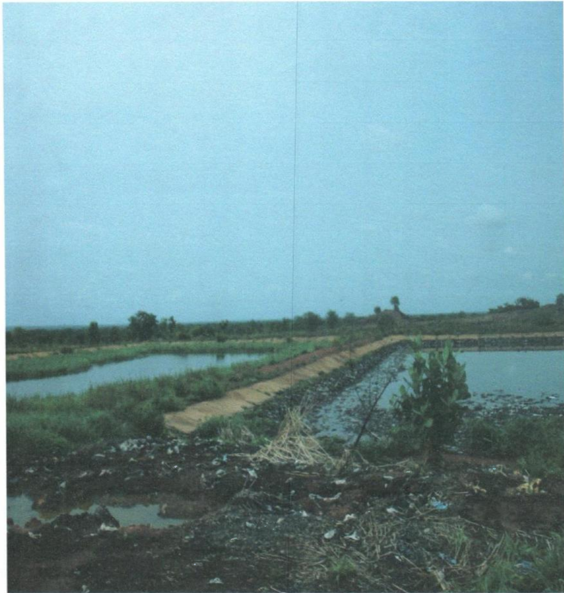
A cross-section of anaerobic and facultative Pond for liquid waste for sludge settlement at the Tamale engineered Sanitary Landfill site.
