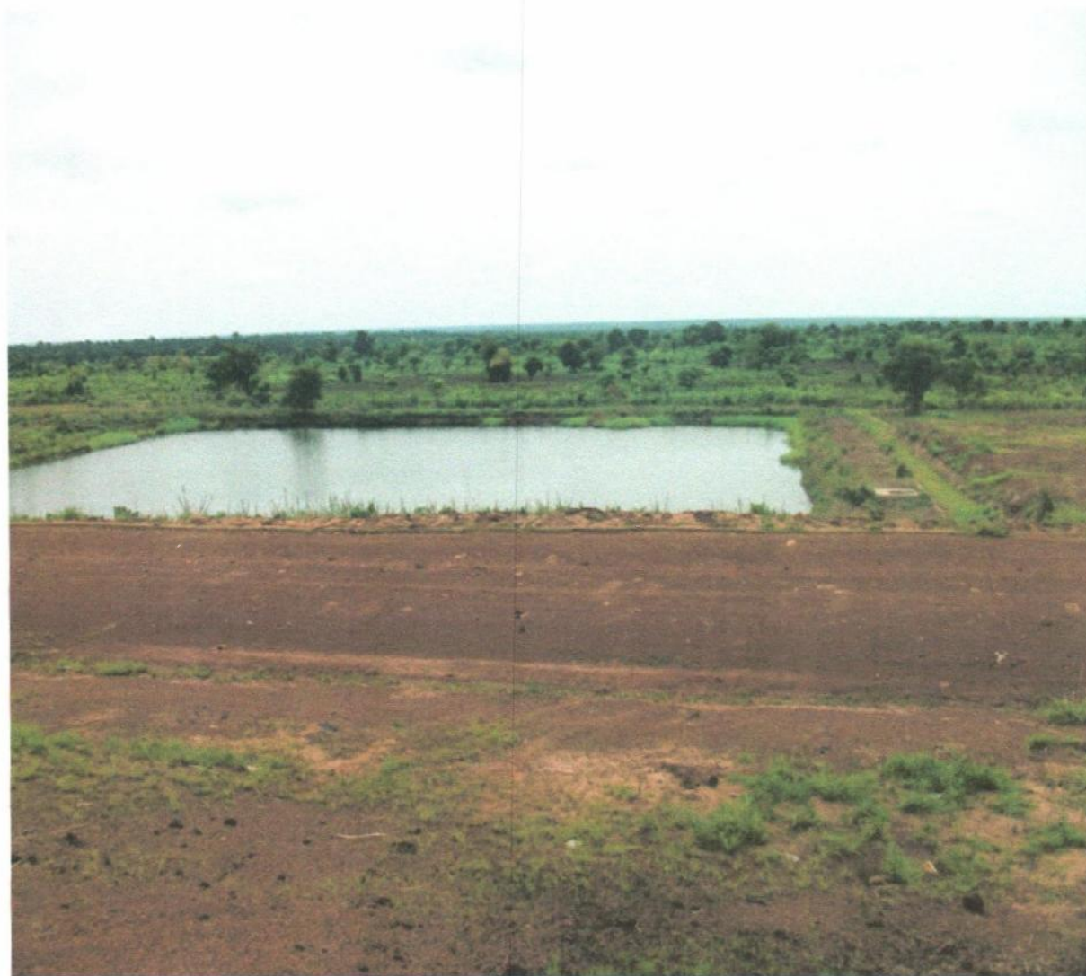
Maturation Pond (Final) where germs are killed to keep the water safe at the Tamale engineered Sanitary Landfill site.
