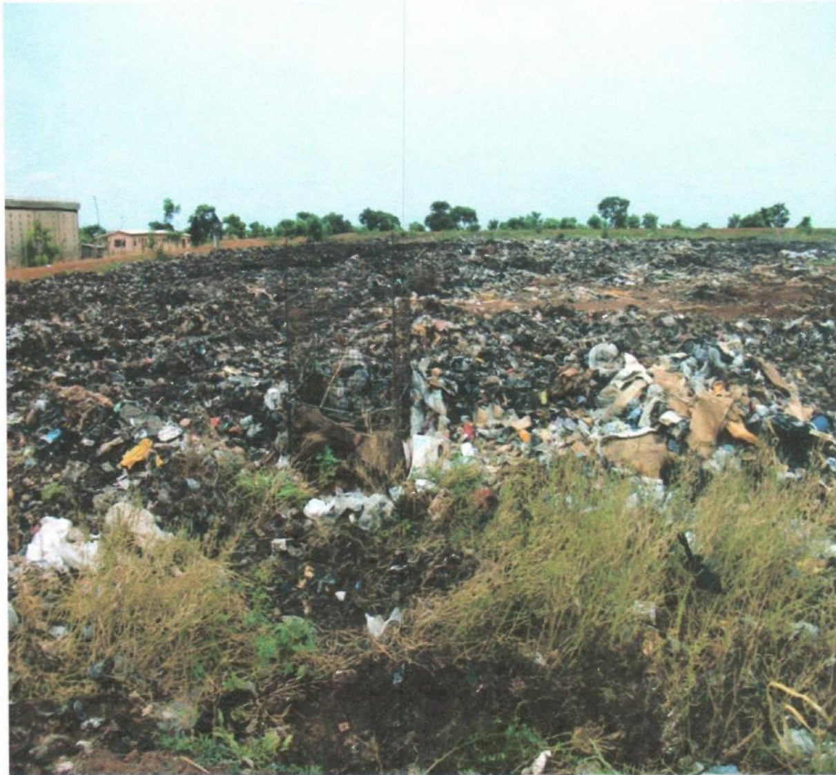
A section of the landfill site with a gas vent through which methane escapes into the atmosphere in the Tamale engineered landfill site.
