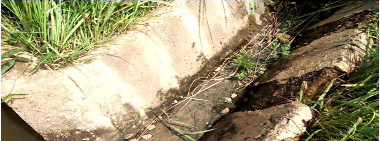
Figure 4a. Broken Down Canals, Daffiama Irrigation Site - Constructed in 2004. Source: Field Survey, November 2010.
