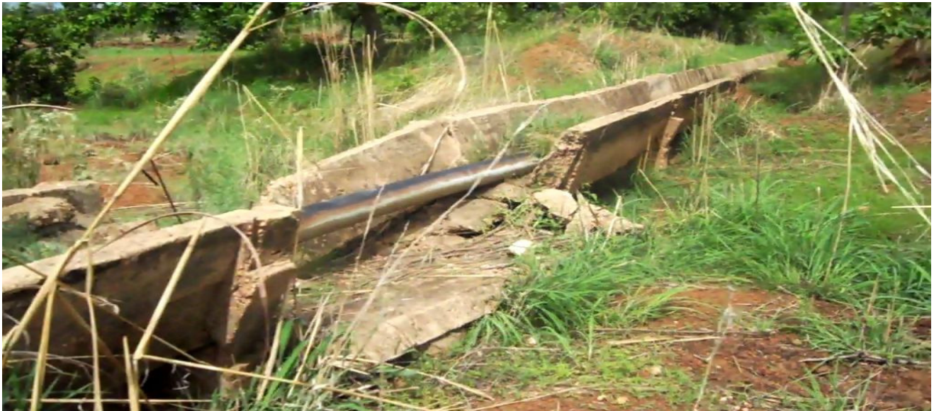
Figure 4b. Broken Down Canals, Daffiama Irrigation Site - Constructed in 2004. Source: Field Survey, November 2010.
