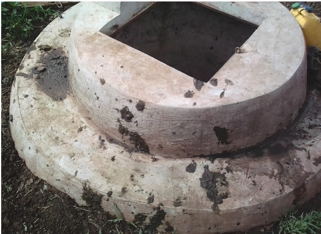
Plate 3: A borehole smeared with cow dung meant for supplying water at Salaga slaughterhouse
