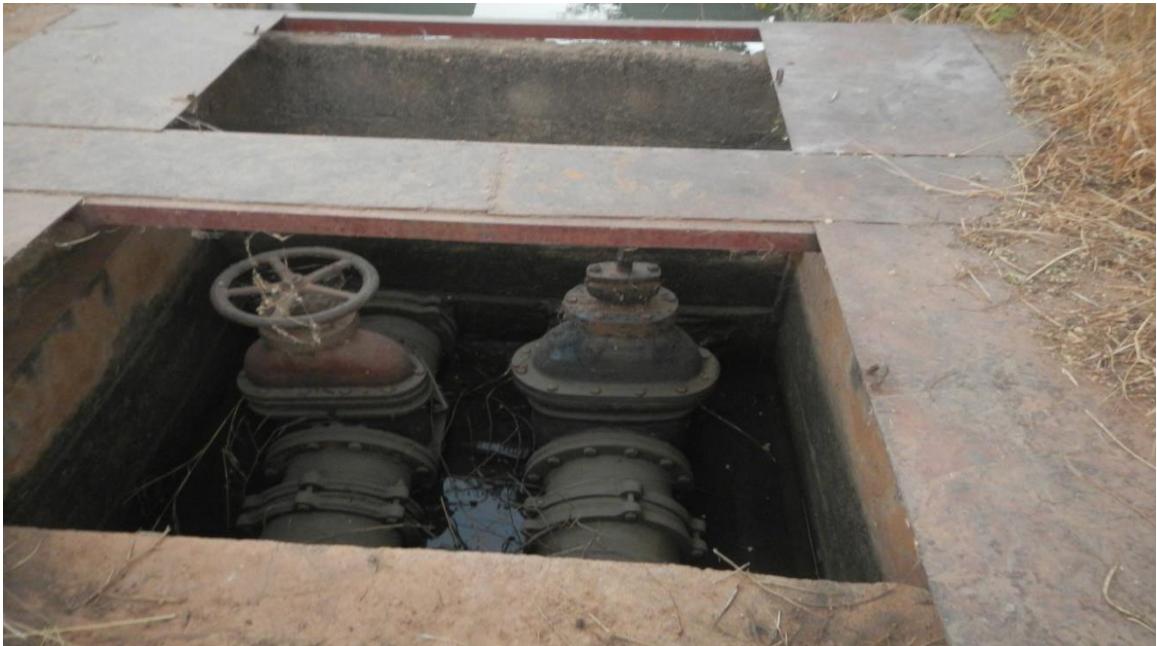
Plate 4.16: Defunct Off-take Valves in Vea Irrigation Scheme
