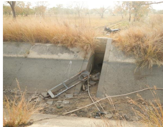
Plate 4.3: Broken Lateral Gates in Tono Irrigation Scheme
