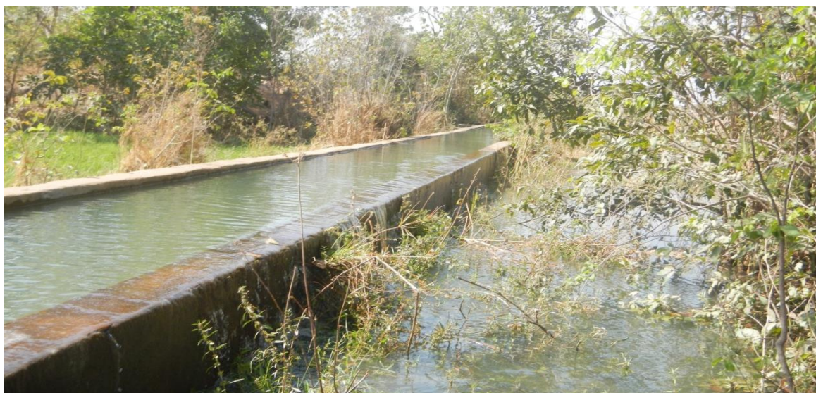
Plate 4.6: Spillage from Canal Causing Waterlogging in the Veia Irrigation Scheme
