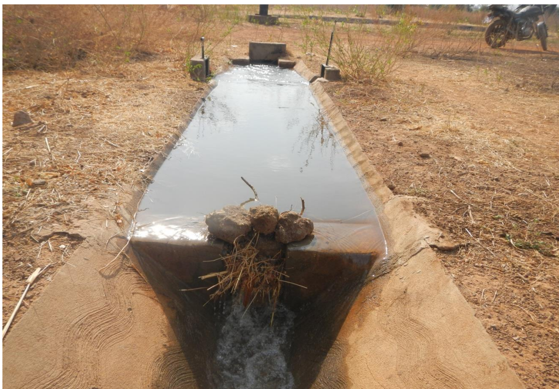
Plate 4.24: Farmers Improvising Check Structure on a Canal Using Sandbags and Stones in the Tono Irrigation Scheme
