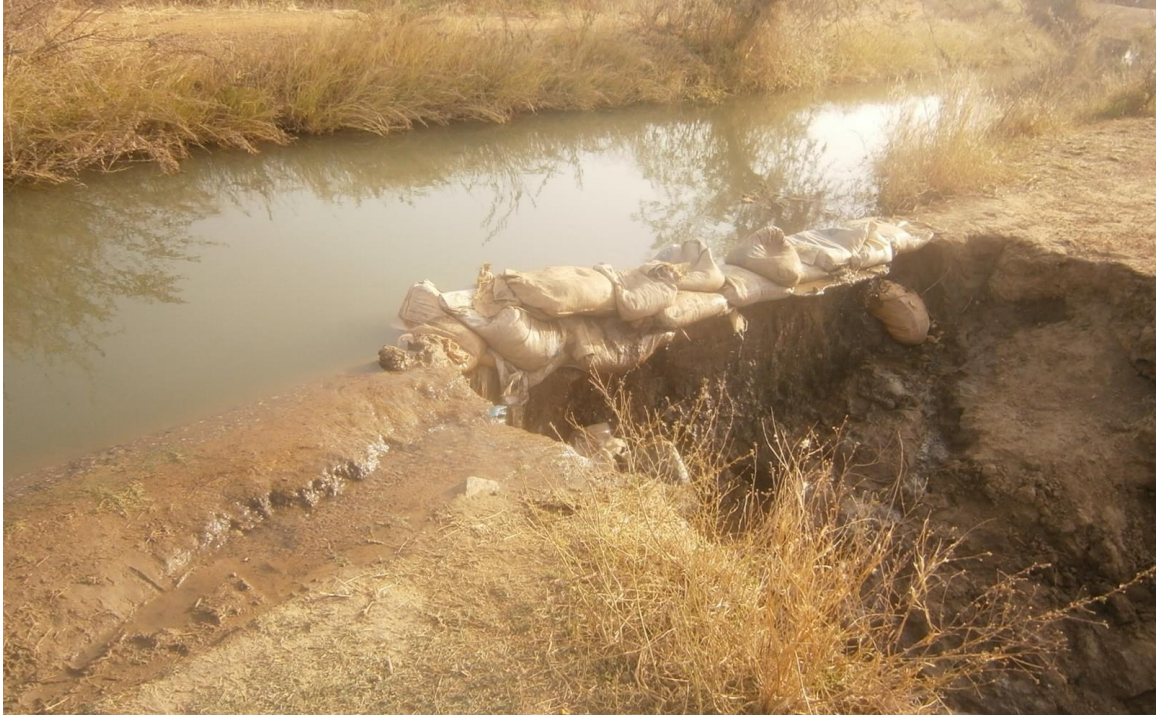
Plate 4.23: Breached Canal Temporarily Repaired With Sandbags by Farmers in the Vea Irrigation Scheme
