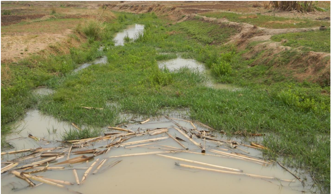
Plate 4.15: Silted and Weedy Main Drain of the Golinga Irrigation Scheme
