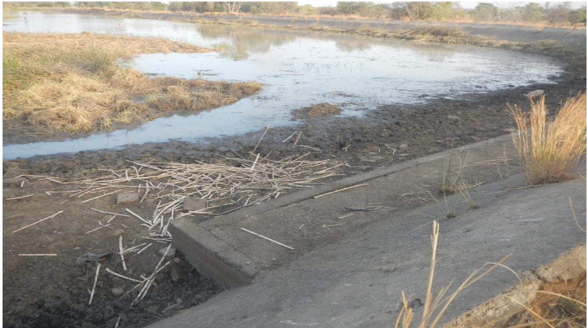
Plate 4.12: Silted and Weedy Night Storage Reservoir in Tono Irrigation Scheme
