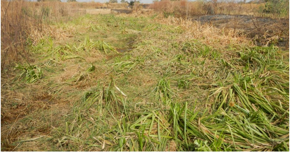
Plate 4.14: Silted and Weedy Primary Drain of the Tono Irrigation Scheme
