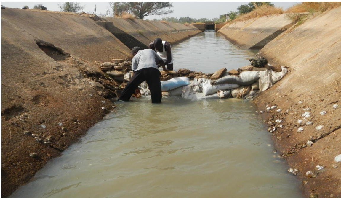
Plate 4.24: Farmers Improvising Check Structure on a Canal Using Sandbags and Stones in the Tono Irrigation Scheme
