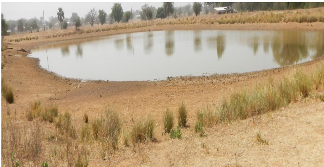
Plate 4.13: Silted Night Storage Reservoir in Vea Irrigation Scheme
