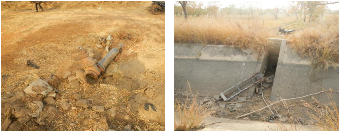
Plate 4.2: Exposed and Broken Lateral Pipes in Tono Irrigation Scheme
