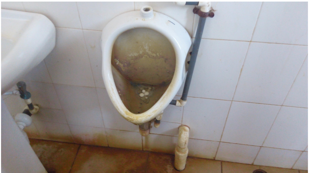
Picture 4.3: Nonfunctioning Urinary
