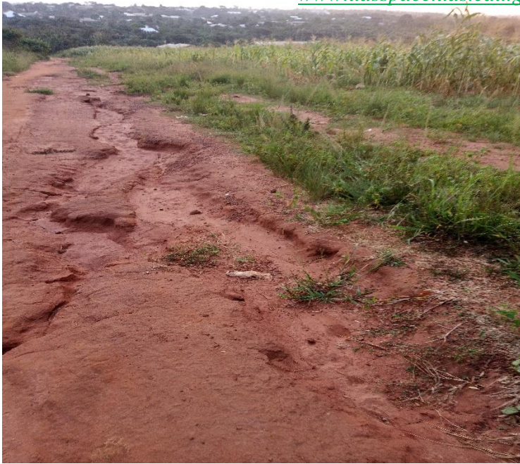
f) Eroded Road Network
