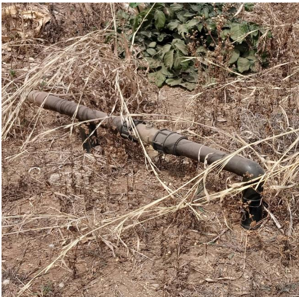
c) Faulty Hydrant Abandoned in the Scheme
