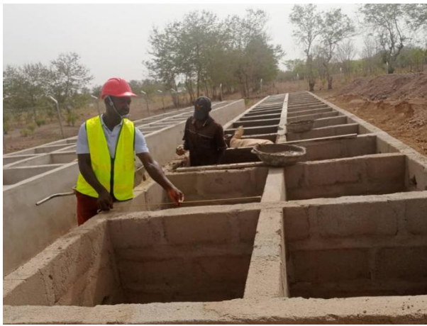
Plate 3.1a: Construction of Microplots
