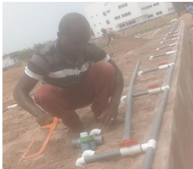
Plate 3.2a: Installation of Sub-Surface Drainage System b. Installation of Irrigation System
