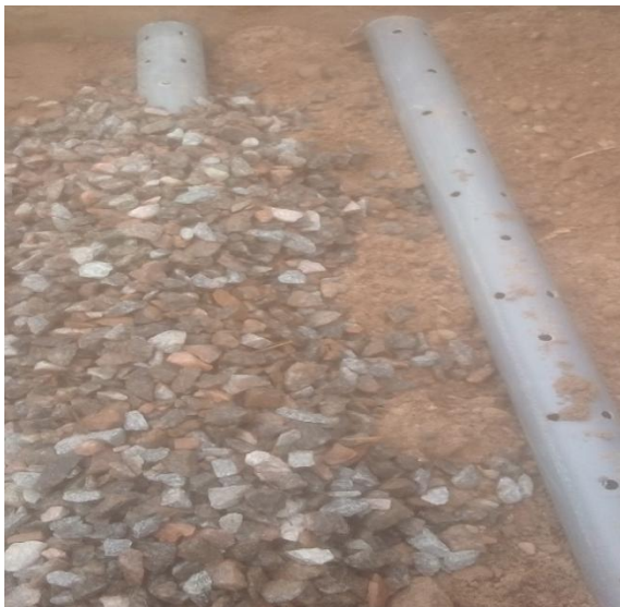
Plate 3.2a: Installation of Sub-Surface Drainage System b. Installation of Irrigation System
